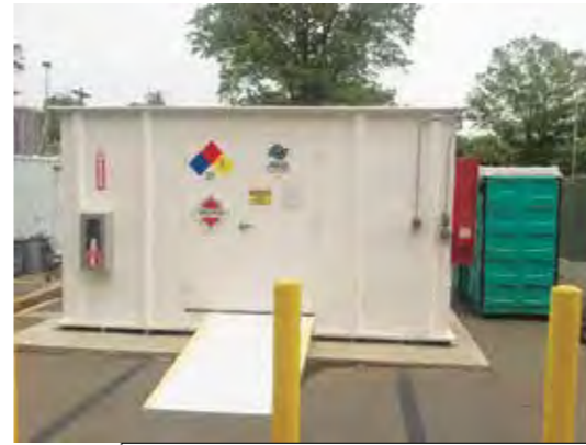
(6) HAZARDOUS MATERIALS STORAGE BUILDING.
